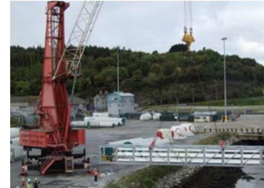
G1 crane placing the pipe bridge across the back of No. 3 jetty as part of the new AFSC terminal project.
