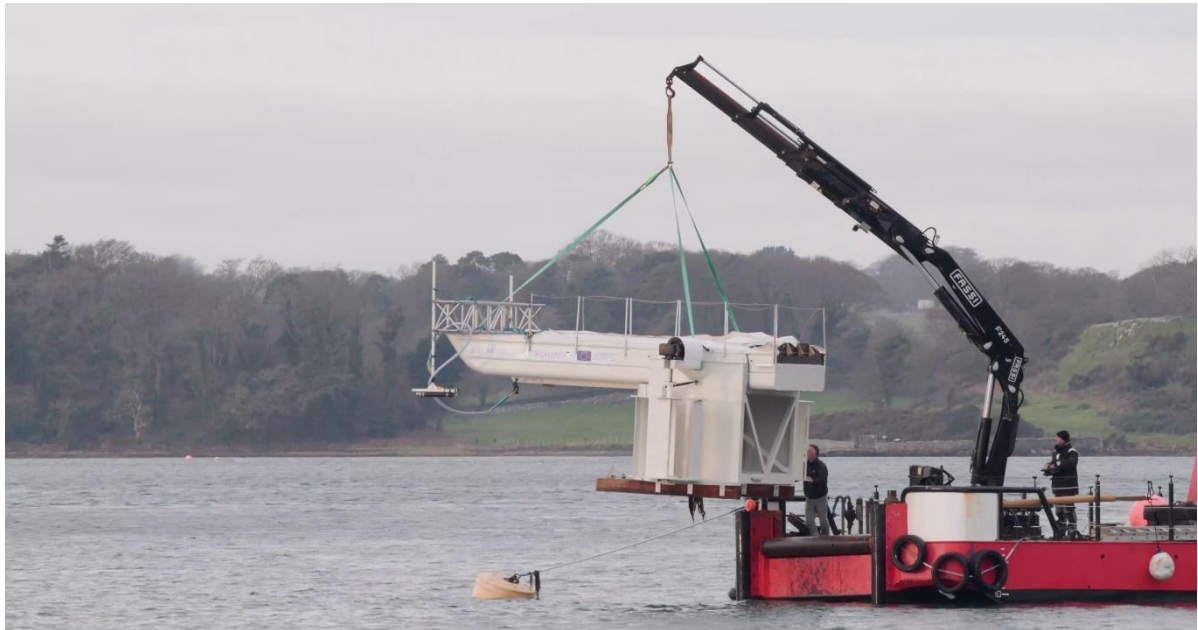
Figure 5 - Deploying the GKinetic CEFA12 to mooring
